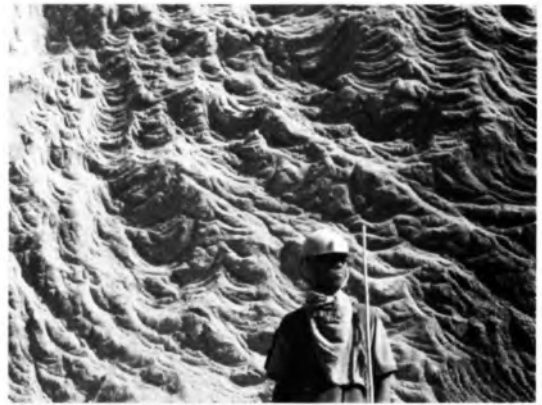
Photo-5 Groves cut by Twin Cutter
