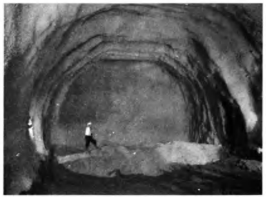
Photo-6 Tunnel excavated by Twin Cutter
